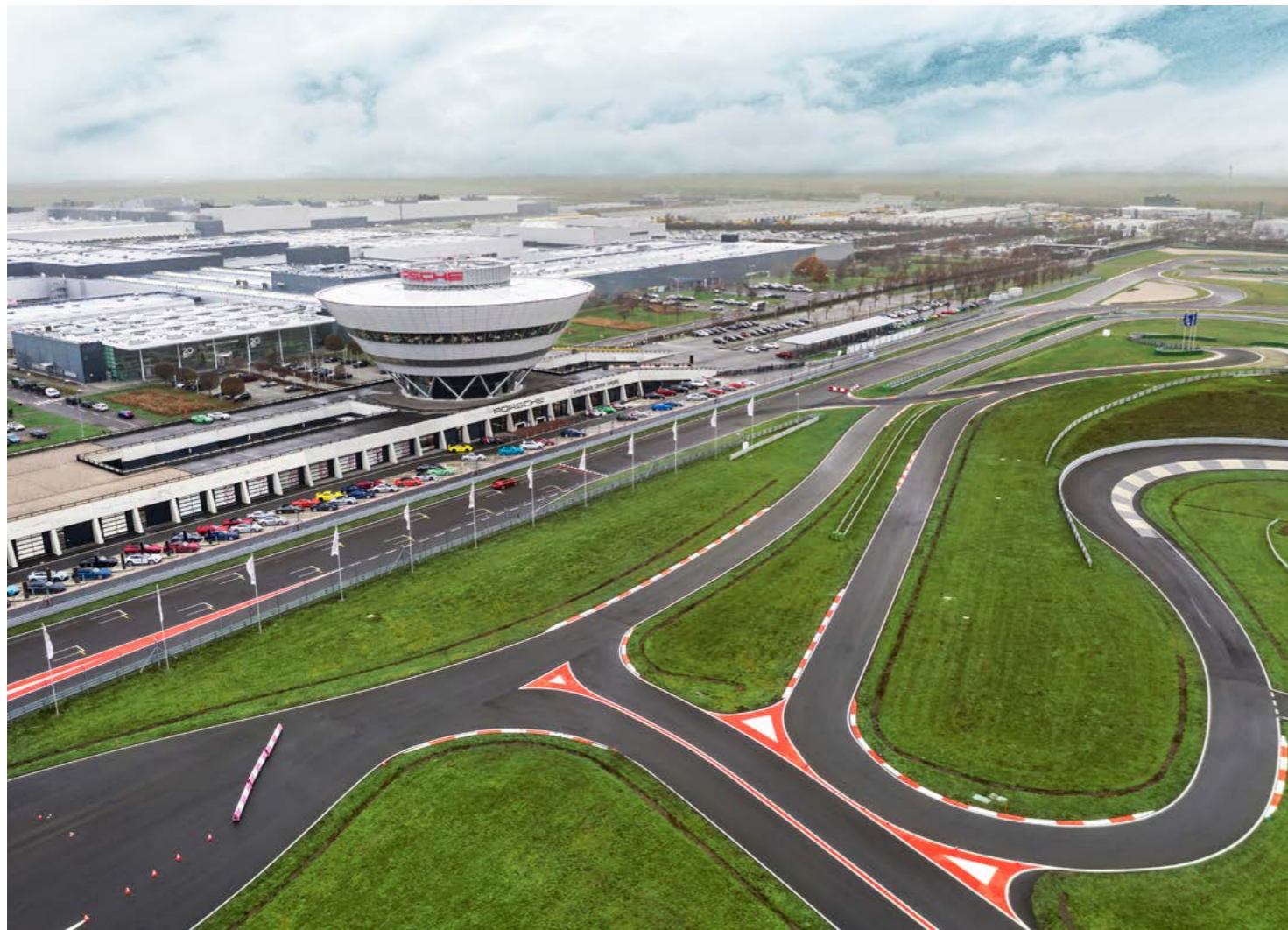
The site at a glance: the Porsche Experience Center in front of the production facilities
